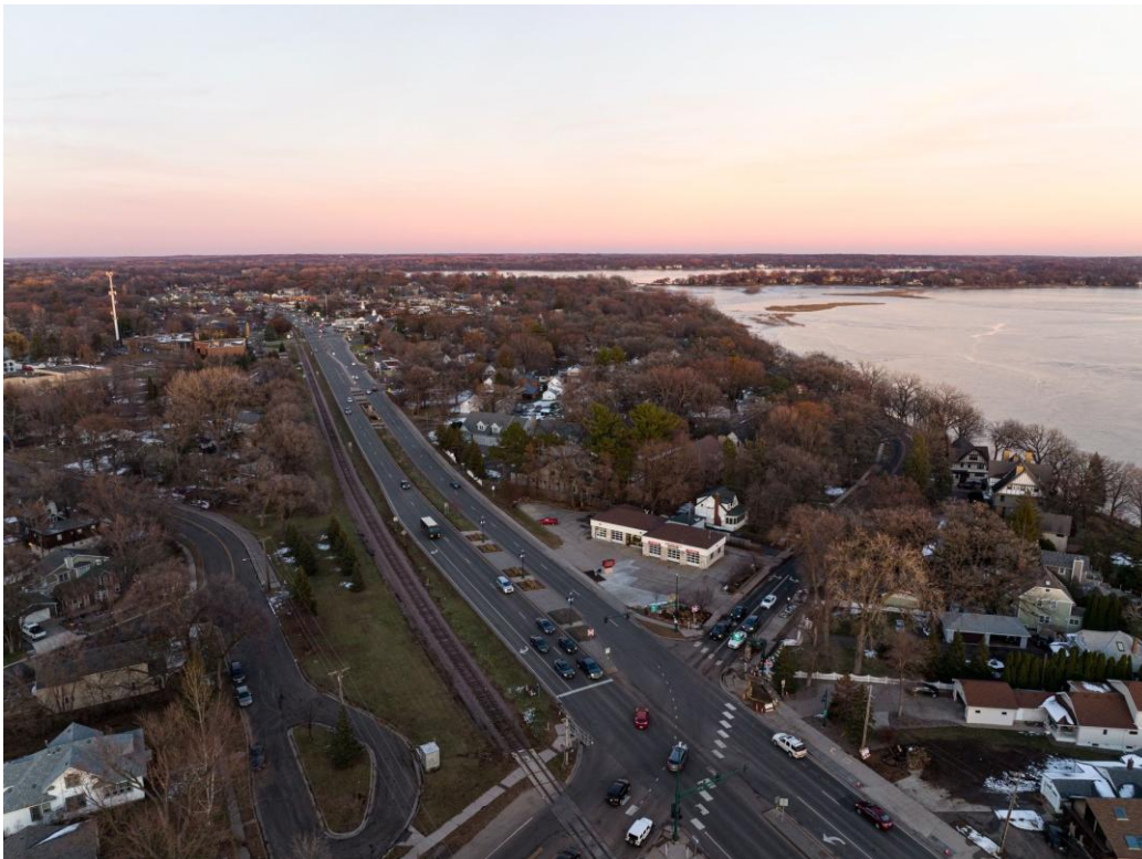
4561 Lake Avenue — Aerial view of building, drive lanes, and monument sign
