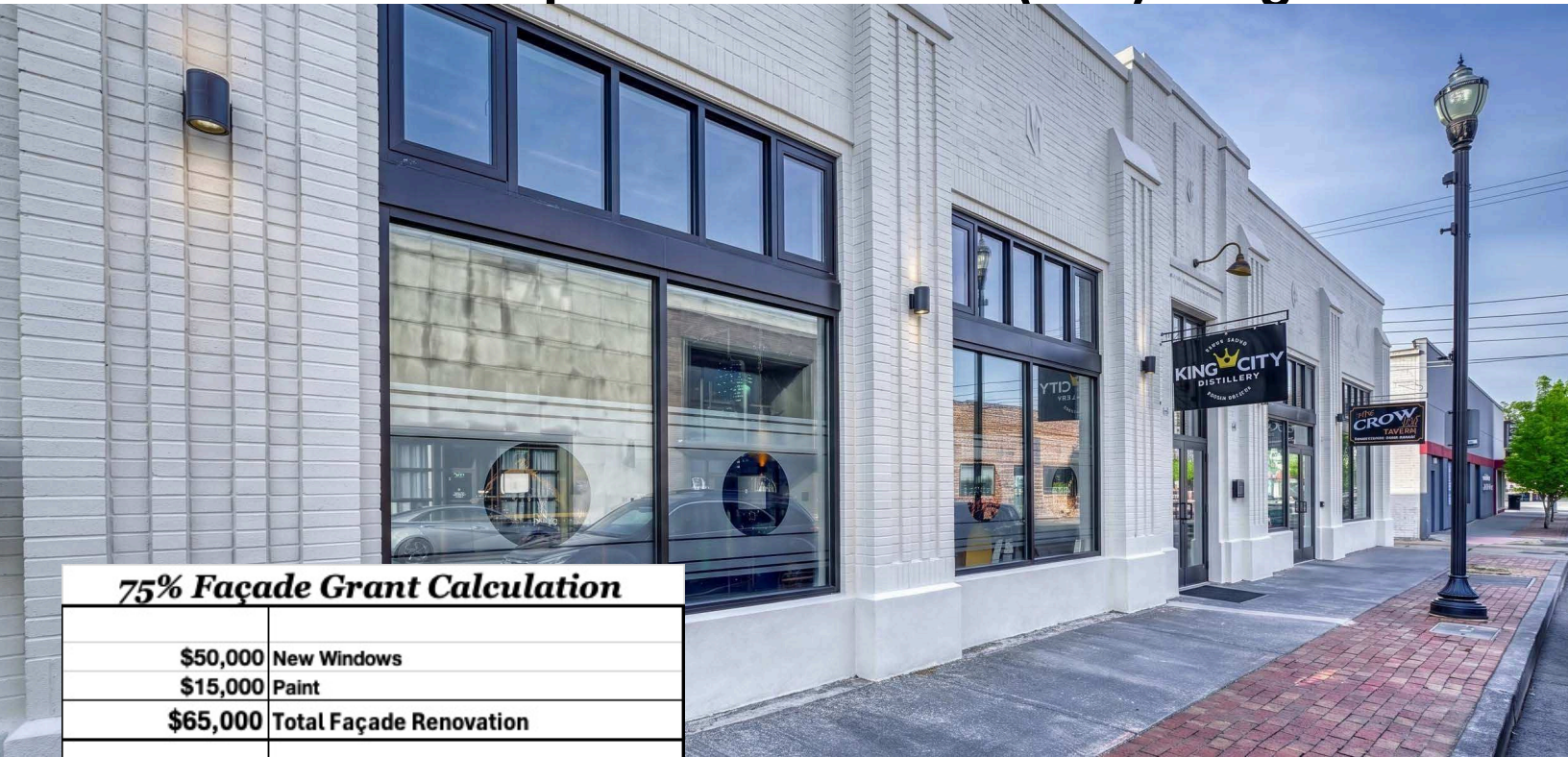
Facade Grant - Potential Renovation
