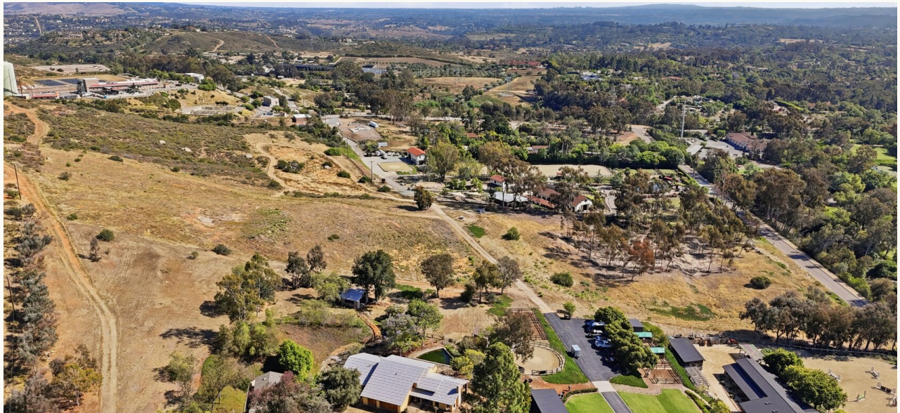
The site set between two established equestrian facilities, with the San Dieguito valley beyond
