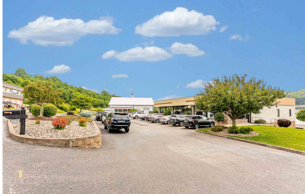
Exterior Front of the Building/Parking Lot.
