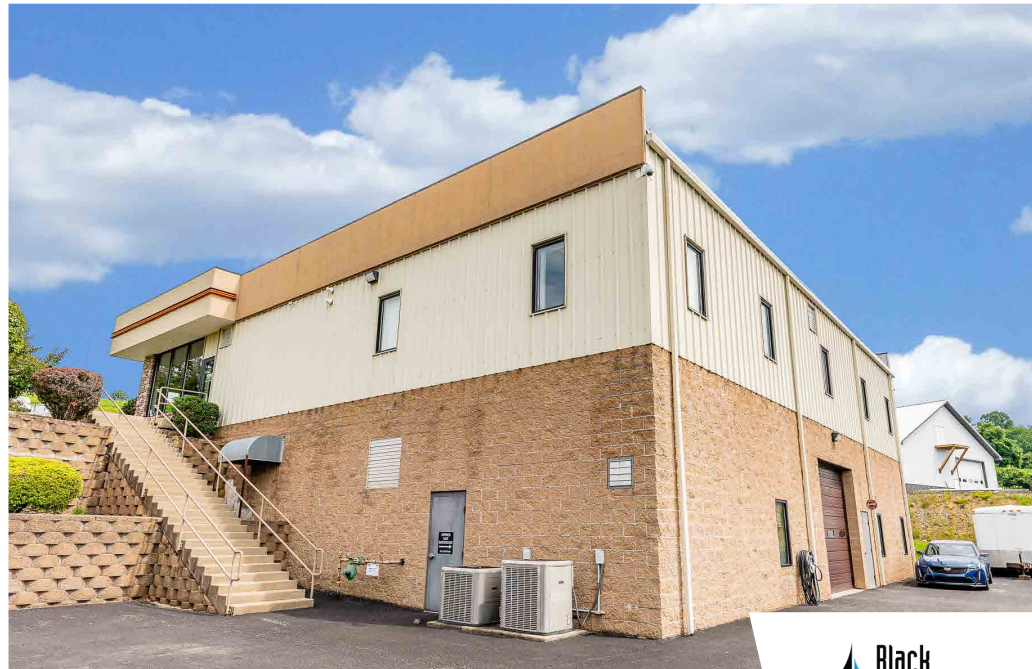
Exterior Back of the Building.
