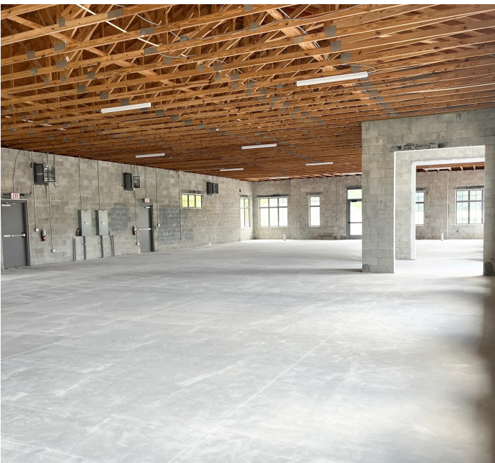
CONCRETE SLAB IN PLACE
