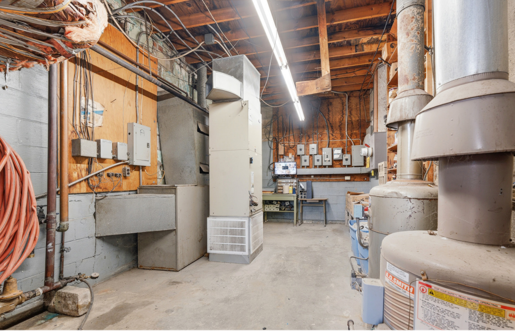
Fay-West Glass Company - Interior.
