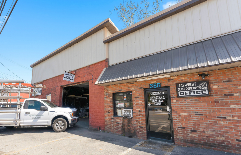
Fay-West Glass Company - Exterior.
