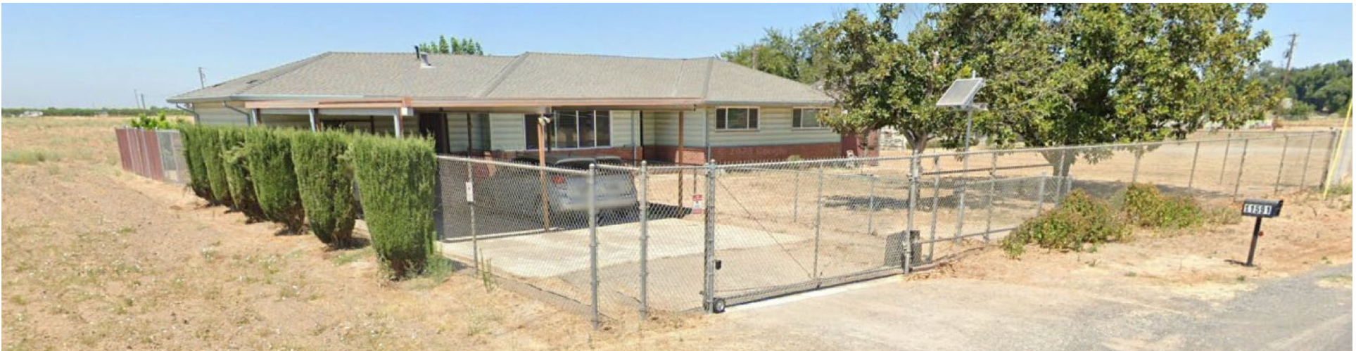
EXISTING RESIDENCES ON PARCEL 191-250-070
