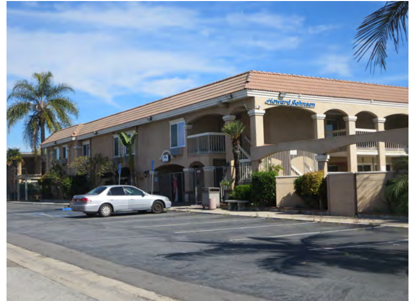
Building A Angle View
