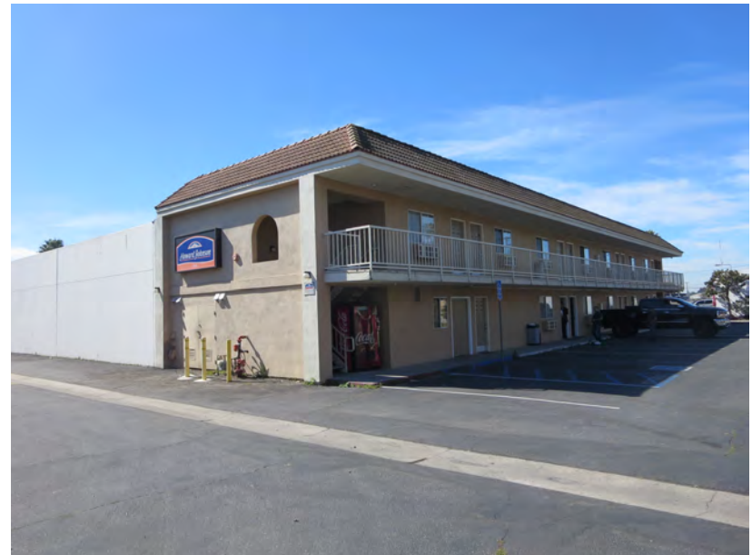
Building B Exterior
