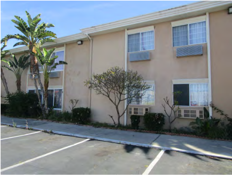
Building A Side Wall
