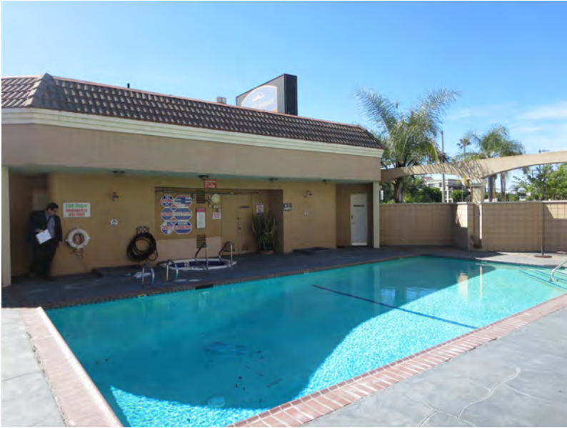
Building C and Pool
