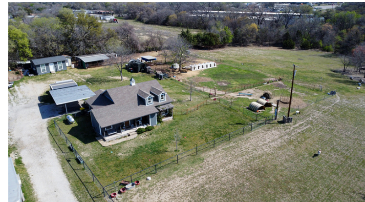
Existing residential improvements offering immediate use or redevelopment potential
