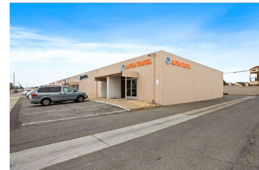
DRIVE AROUND ACCESS
