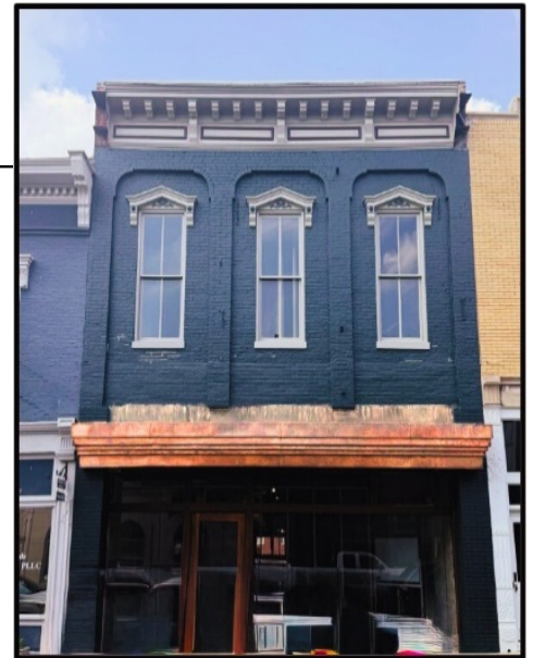
Exterior: 34 FT Main Street Frontage
