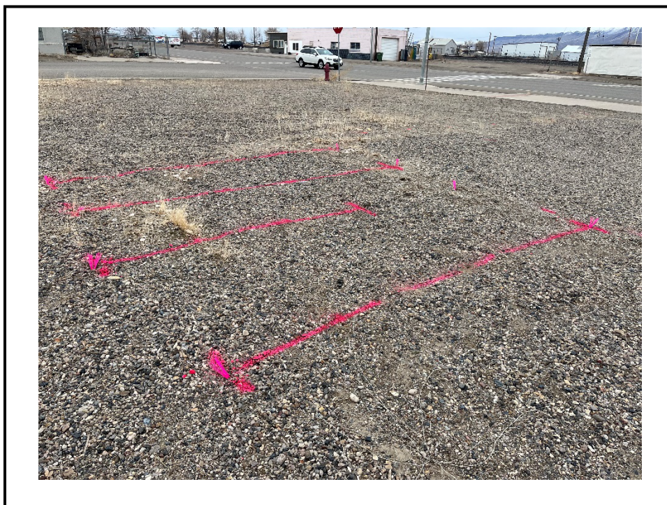
Photograph 2: View of four suspect USTs located in the northern portion of the Site.
