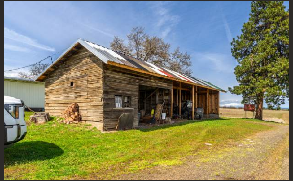
STORAGE & TOOL SHED- 3 BAY
