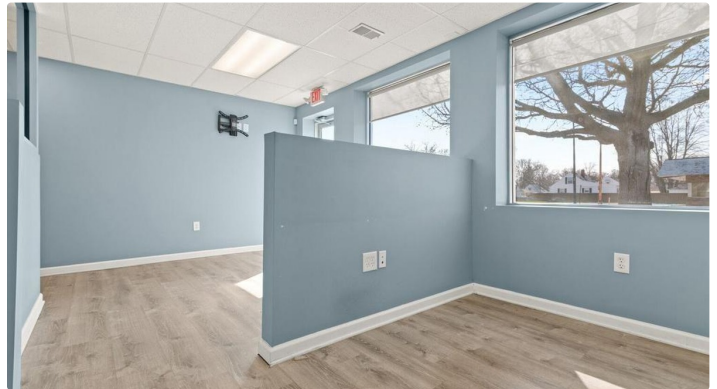
CONFERENCE / OFFICE — GLASS PARTITION
