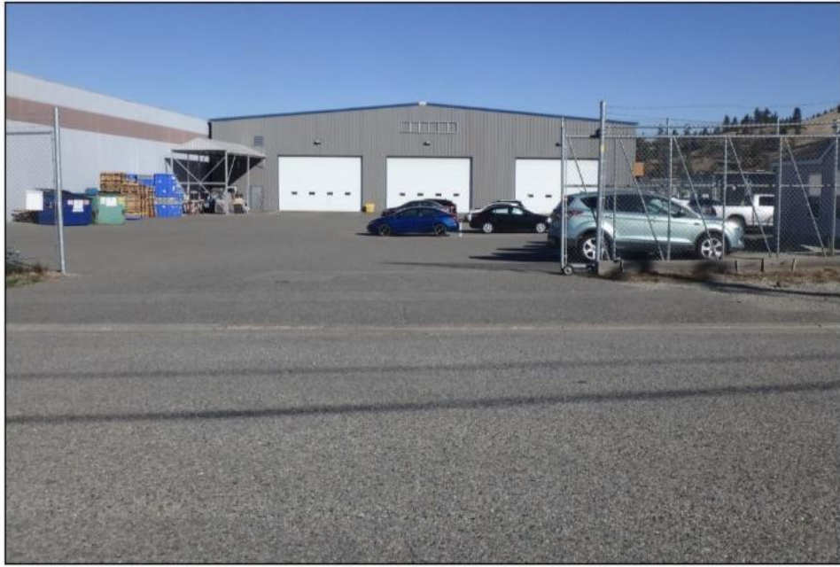
South elevation and parking lot, viewed from Carion Road.
