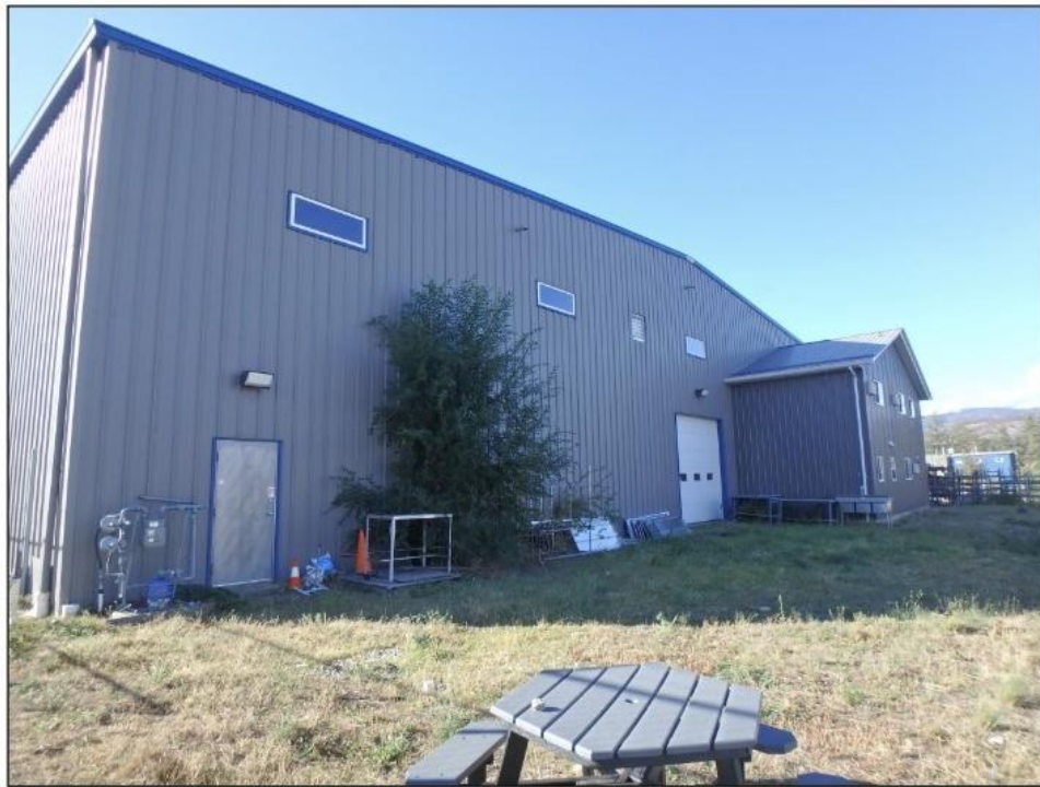
North elevation of the building, viewed from the northeast corner of the property.
