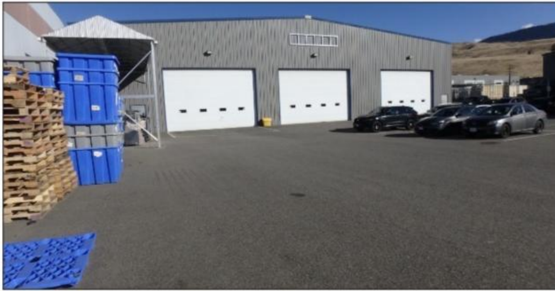
Front of building with grade-level overhead doors and paved parking / yard area.
