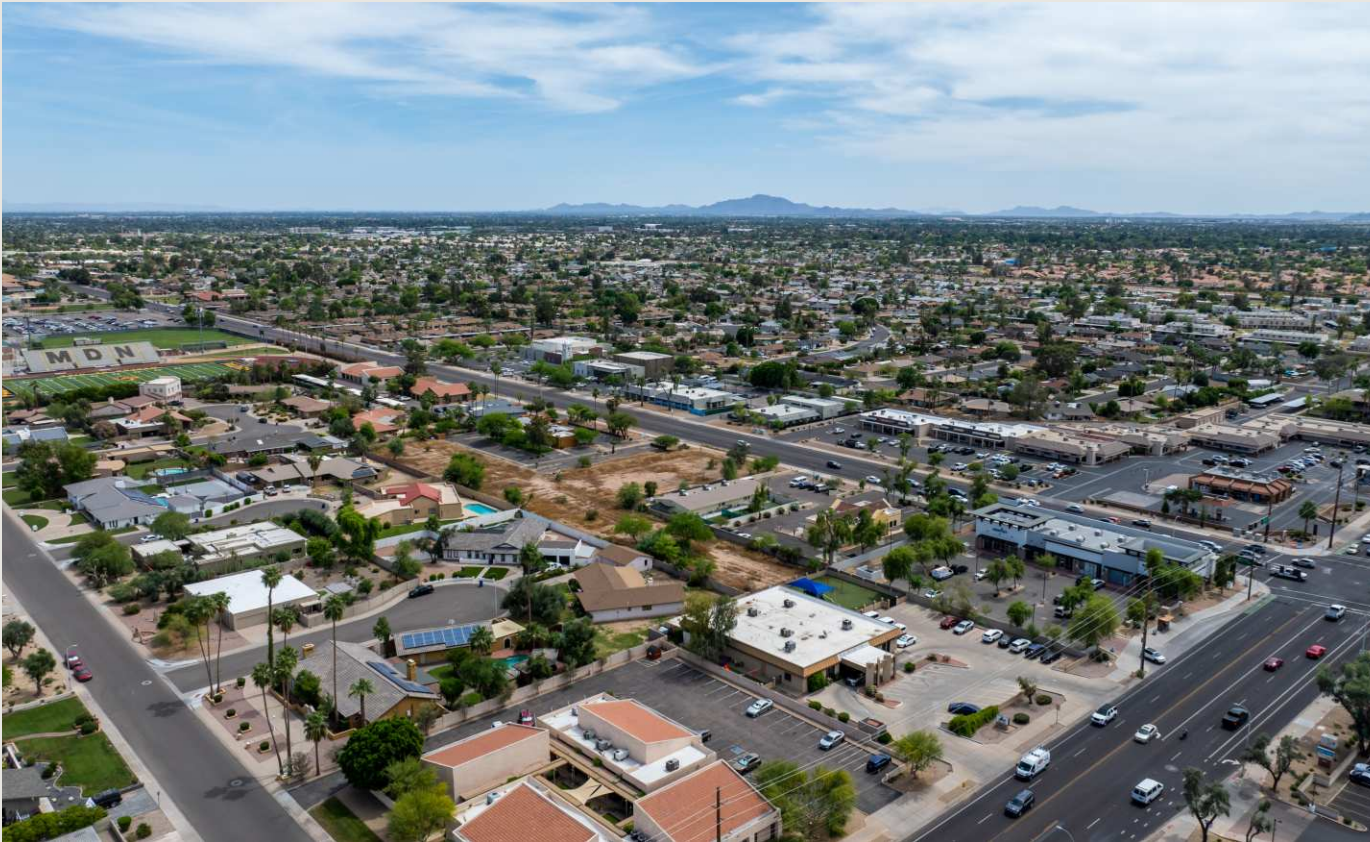
Fig. 01 • Subject site looking southeast
