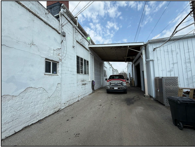
Delivery access through alley. Overhead door (13'7" x 14")
