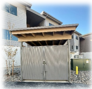
Enclosed shared trash dumpster
