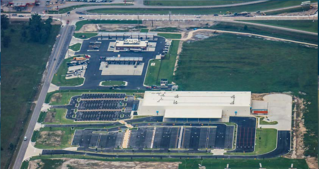
Amazon Distribution Facility
