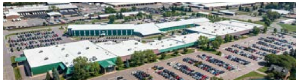
Menards, Inc. employs thousands across the nation and 300+ locally at their headquarters.
