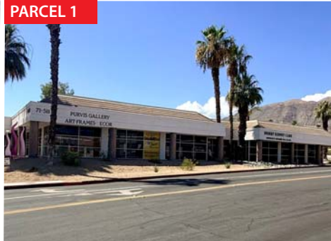
Mirage Business Mall Bldg Size: 12,900 SF APN: 684-232-019
