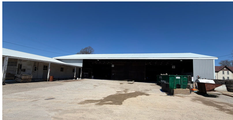
Storage Building #1 | With 225-amp, 3-phase power
