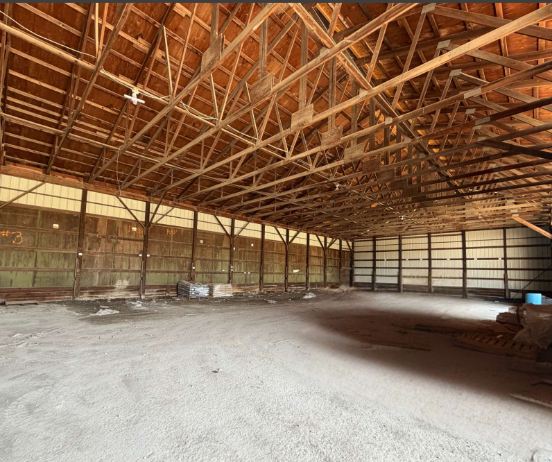
Storage Building #1 Interior
