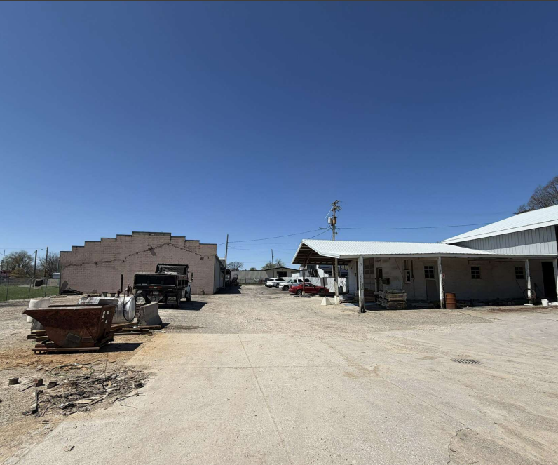
Multiple Storage Buildings
