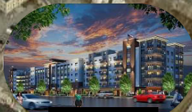
Station Lofts New Broad St 180 Units
