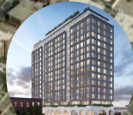
157 Westchester Ave 190 Residential Units Mixed Use
