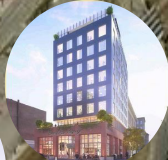
36 Broad St 36 Units Mixed Use *In Construction
