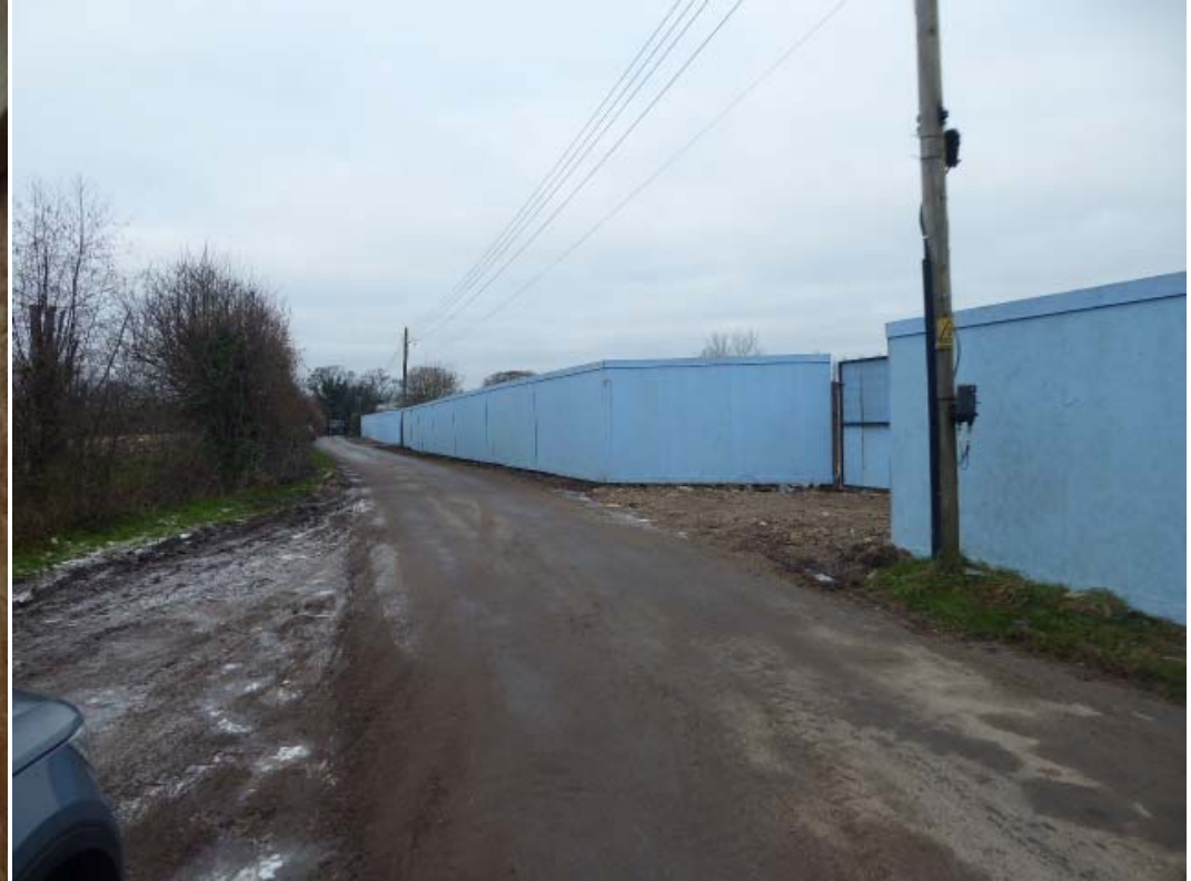
FRONTAGE OF SITE TO MARLE PLACE ROAD - JANUARY 2025
