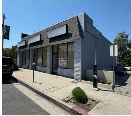
Front and east side of property
