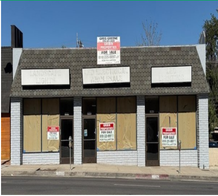
Front of Building
