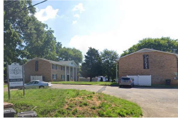
5 205-207 DOUGLAS STREET Cartersville, GA 30120
