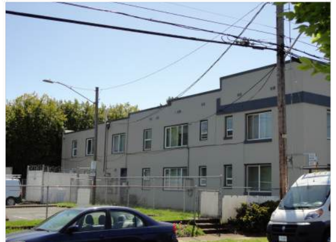
Exterior Parking Lot View
