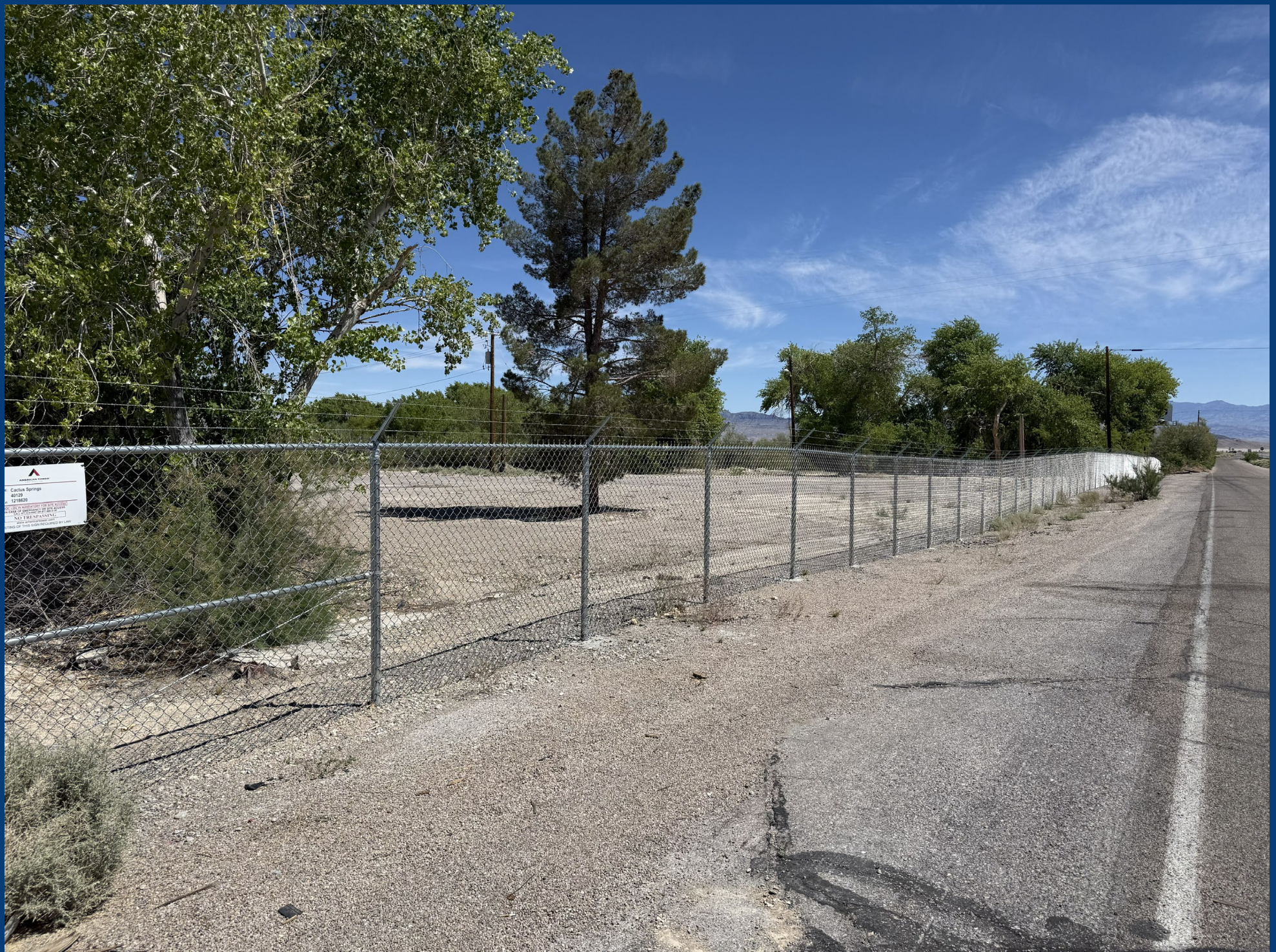
FRONTAGE FENCE – LOOKING SOUTHEAST
