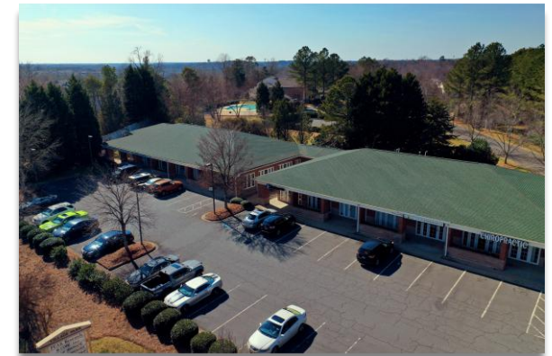
OFFICES AT VILLAGE PARK
