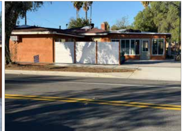
Back Part Of Existing Home
