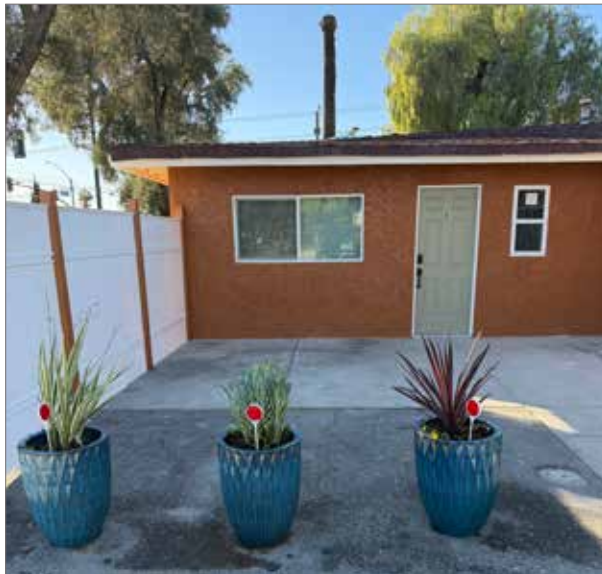
Entrance To Back Unit/Studio
