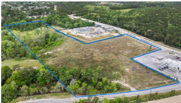
VIEW OF PROPERTY LOOKING NORTH
