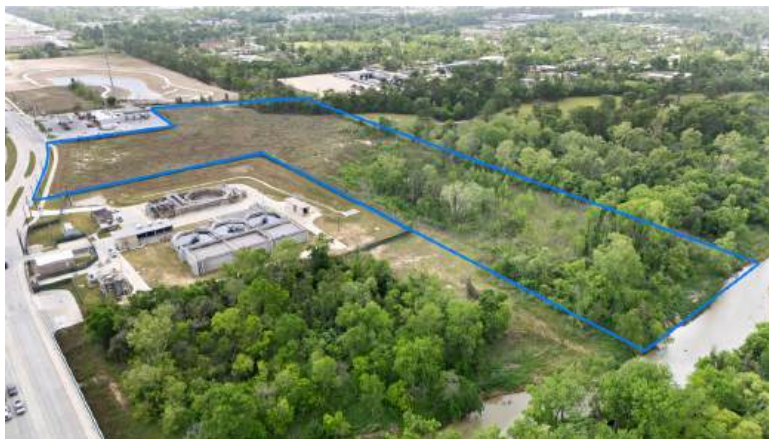
VIEW OF PROPERTY LOOKING SOUTH
