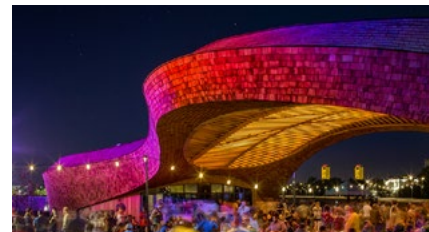
The Barn (Completed) Designed by Dutch designer Jerry van Eyck and his urban design and landscape architecture firm !Melk, The Barn provides 9,100 SF under canopy shade while patrons enjoy craft drinks by Drake's Brewing.
