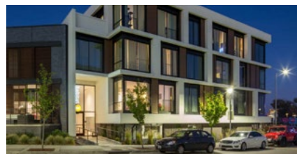
Habitat Apartments - 96 Units (Underway) The Habitat Apartments frame the 4 corners of Garden Park and are steps away from a 1-mile long stretch of West Sacramento's Riverwalk. Opening June 2026.
