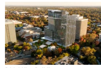
DGS Office Building (Underway) 20 stories and ± 838,000 SF will include office, assembly, parking, retail, and commercial food service space.
