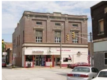
Storefront scale, façade rhythm and proportion have been compromised.
