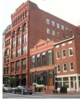
Historic windows have been repaired. New windows on infill structure harmonize with old.
