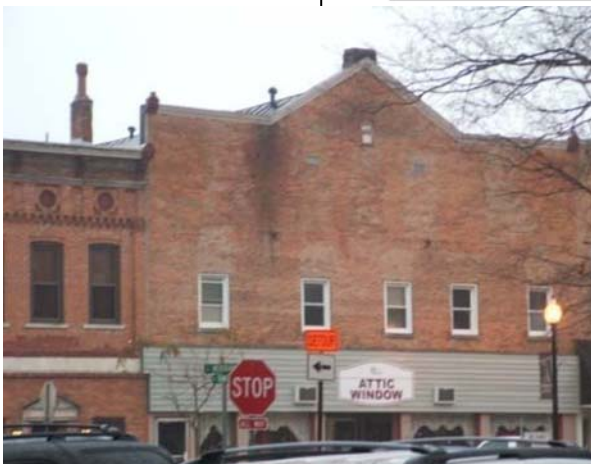
Removing windows eradicates character definition of a building.
