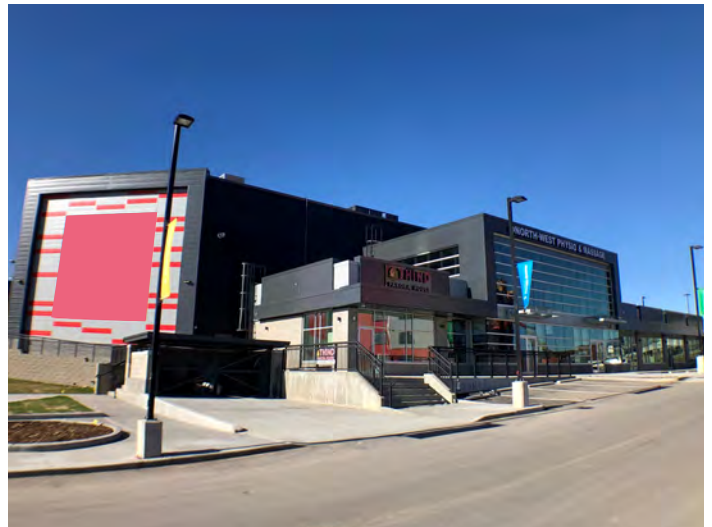
Building U - (Leased)
