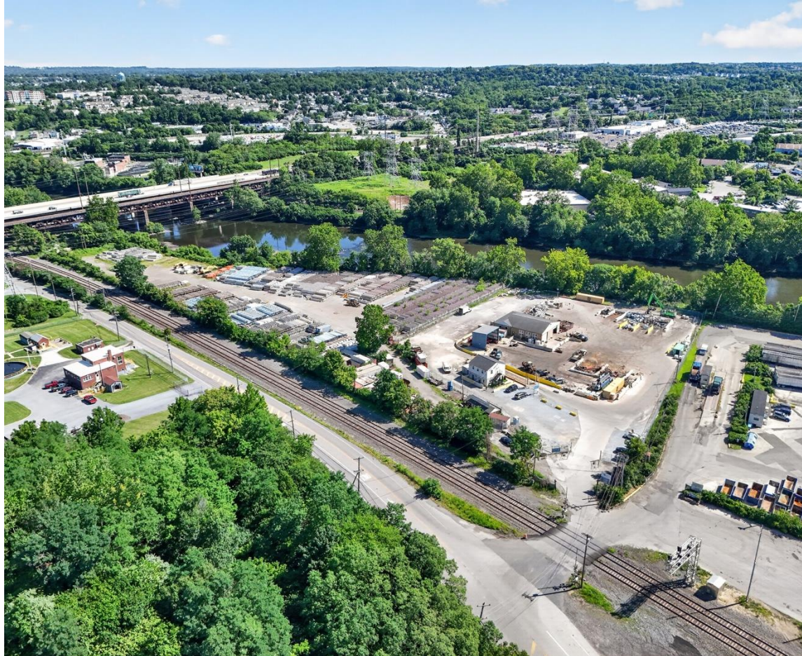
RIVER ROAD FRONTAGE
