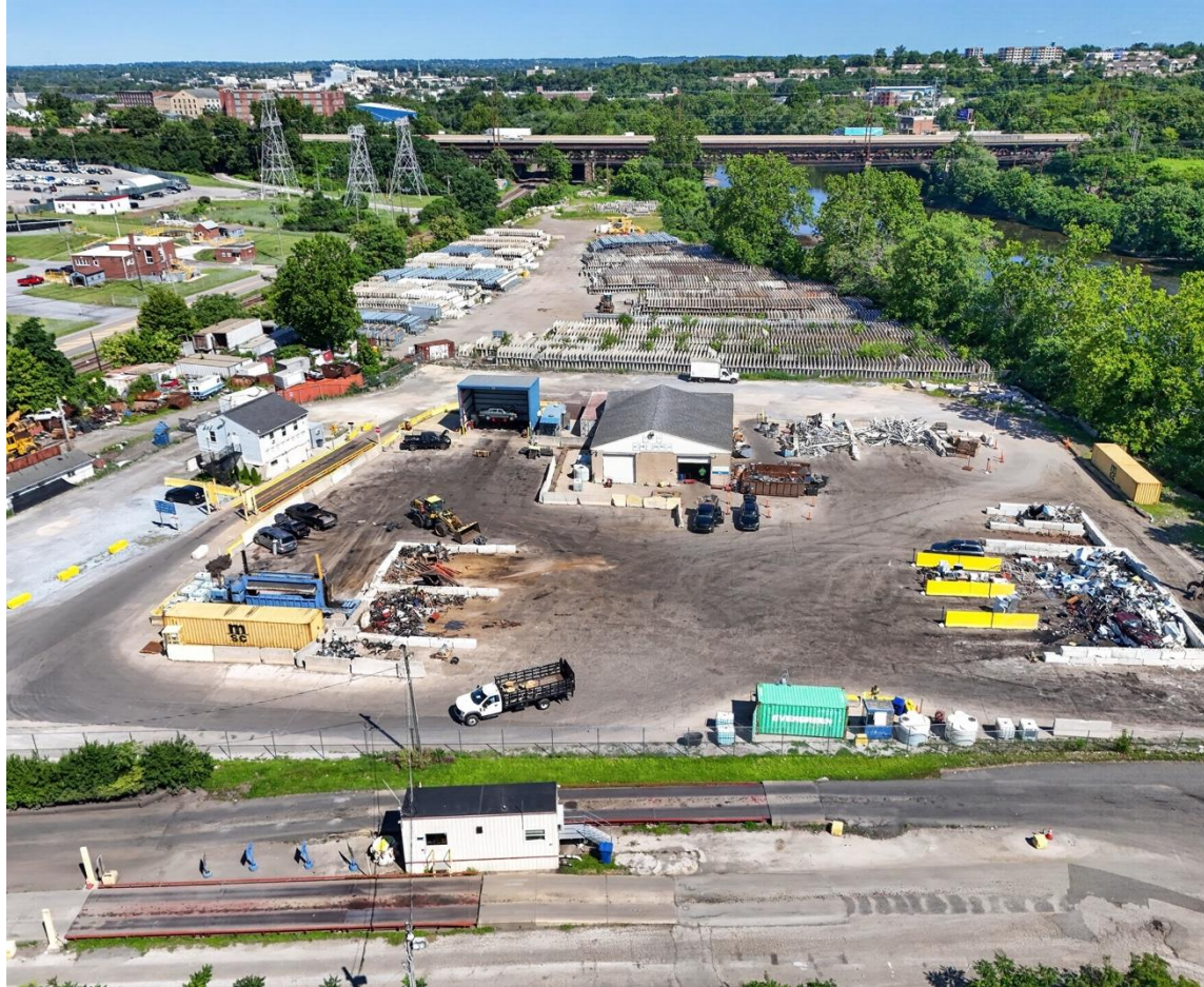
RIVER ROAD FRONTAGE
