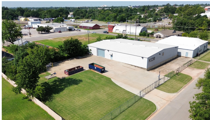
Aerial Overlooking Yard and Warehouses
