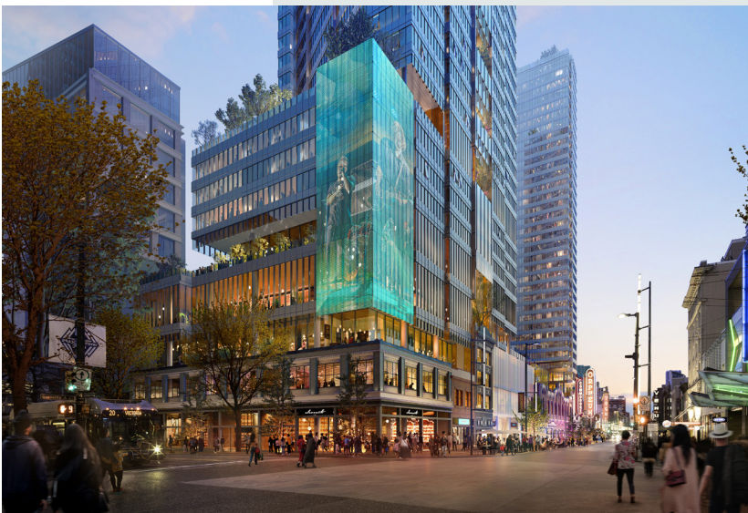
Northwest corner of the project, facing southeast; retail and hotel podium
