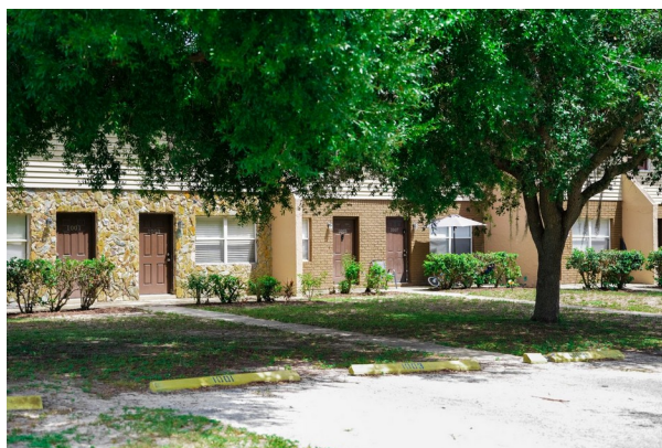
Units 1001-1007 — front elevation, close-up
