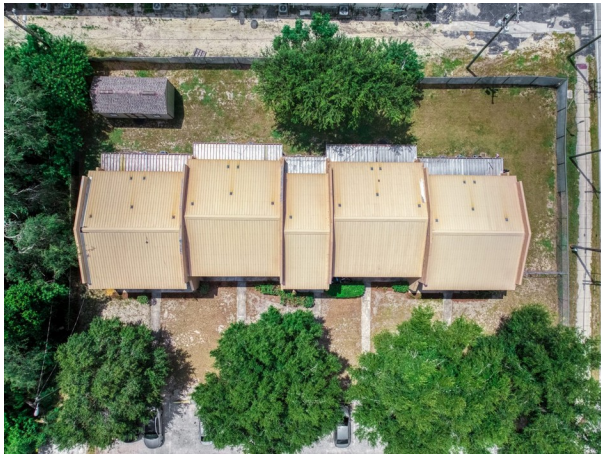
Overhead view — 1000 S Lake Anoka Blvd building
