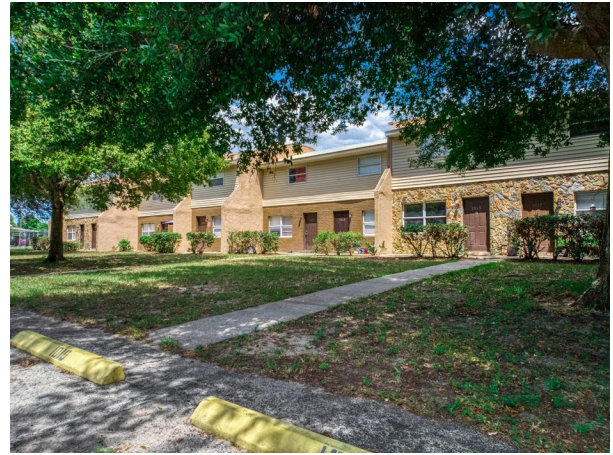
Units 1011-1017 — front elevation, alternate view
