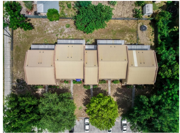
Overhead view — 1001 S Lake Anoka Blvd building
