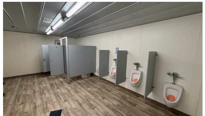
Newer M/ F Restrooms
