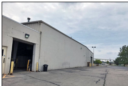
Eastern Elevation - Supply Warehouse
