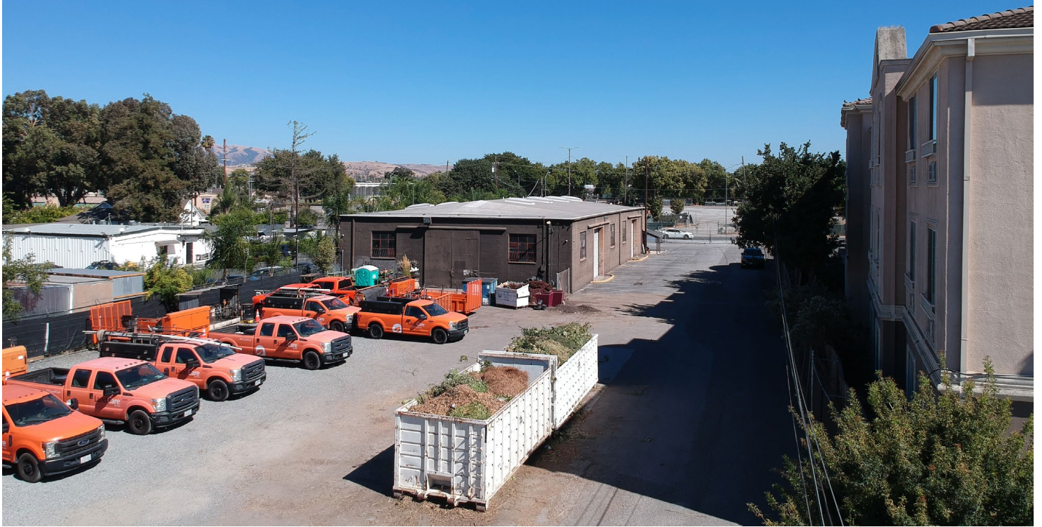
Rear View of the ±7,200 SF Building
