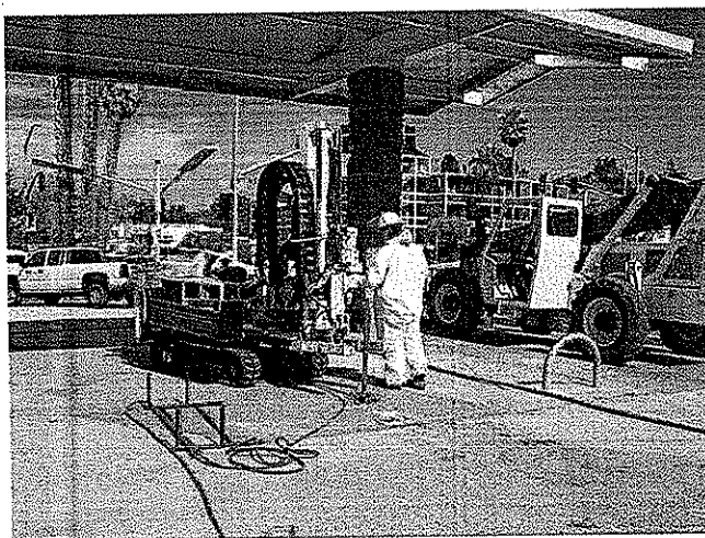
Track mounted DPT injection at former pump island
