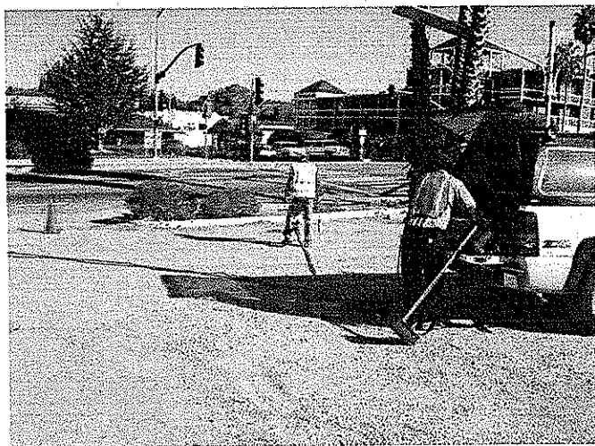
Private utility locator sweeps the site with GPR, pre-injection
