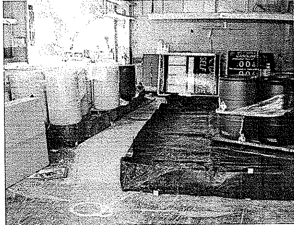
Hydrogen Peroxide and Acidified Iron stored in the service bay in separate secondary containment areas
