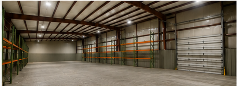
WAREHOUSE - GRADE LEVEL DOOR
