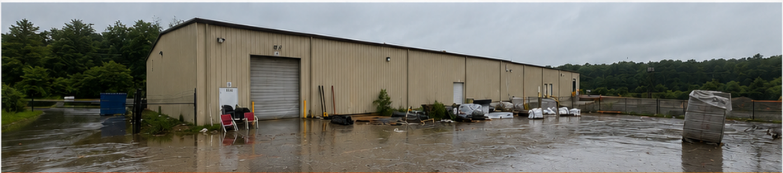
EXTERIOR - LAY DOWN YARD & LOADING AREA
