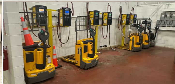
EXISTING CHARGING AREA
