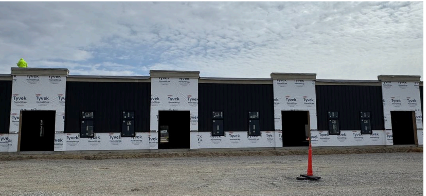
Current Construction (March 2026)
