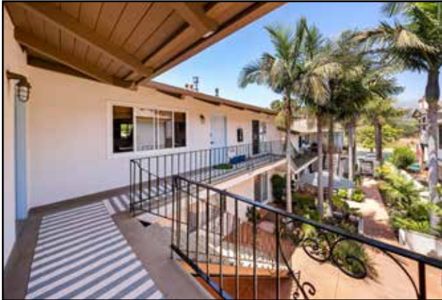
View of Courtyard from Upper Level Walkway
