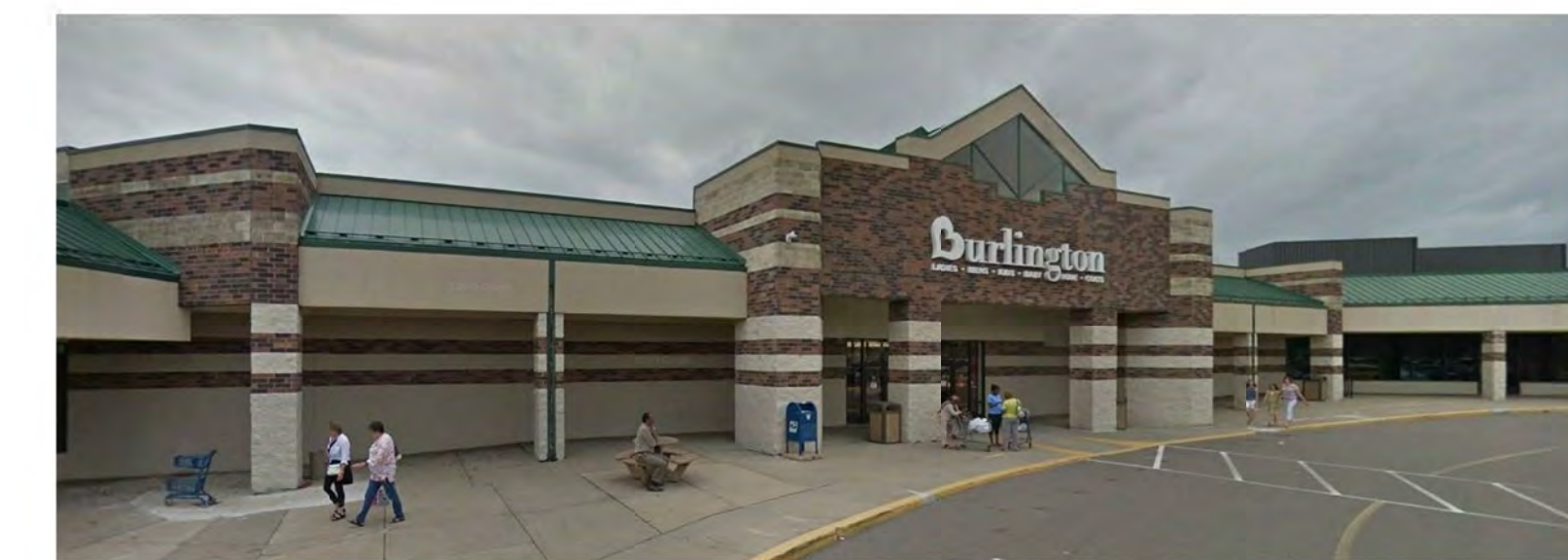
EXISTING STOREFRONT ELEVATION - SOUTHEAST CORNER
