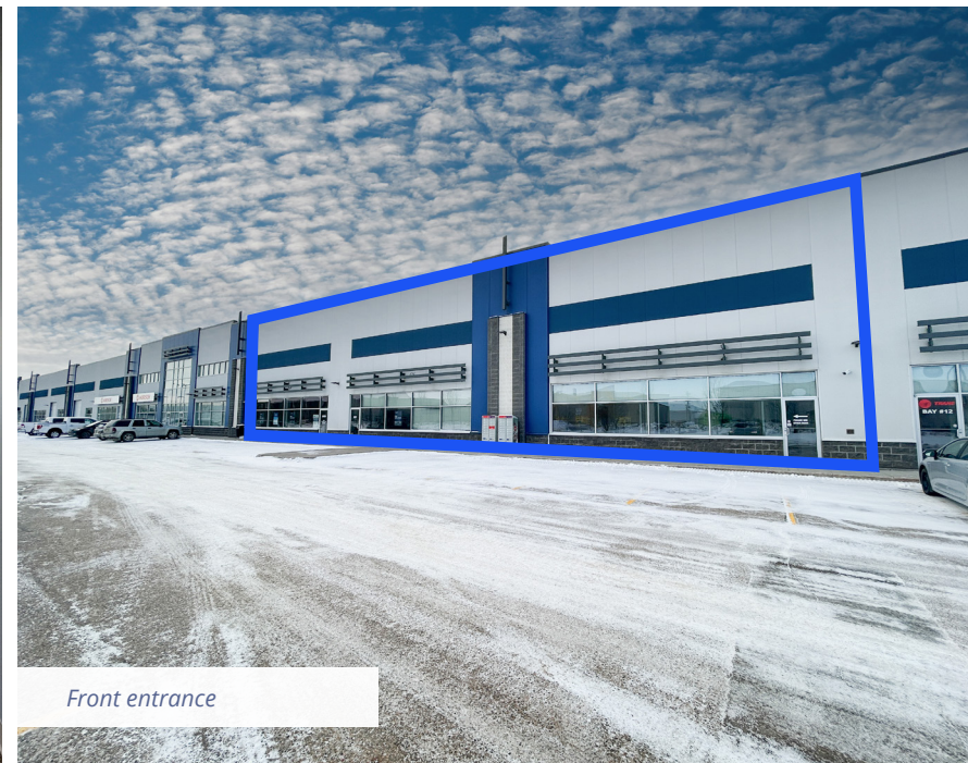
Dock and grade loading
