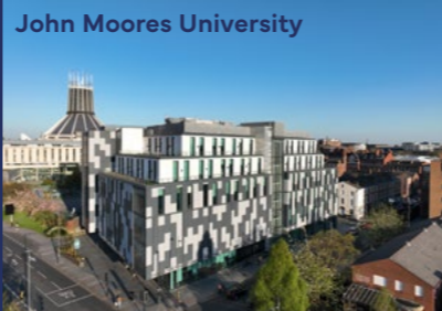
Adjacent Student Accommodation
