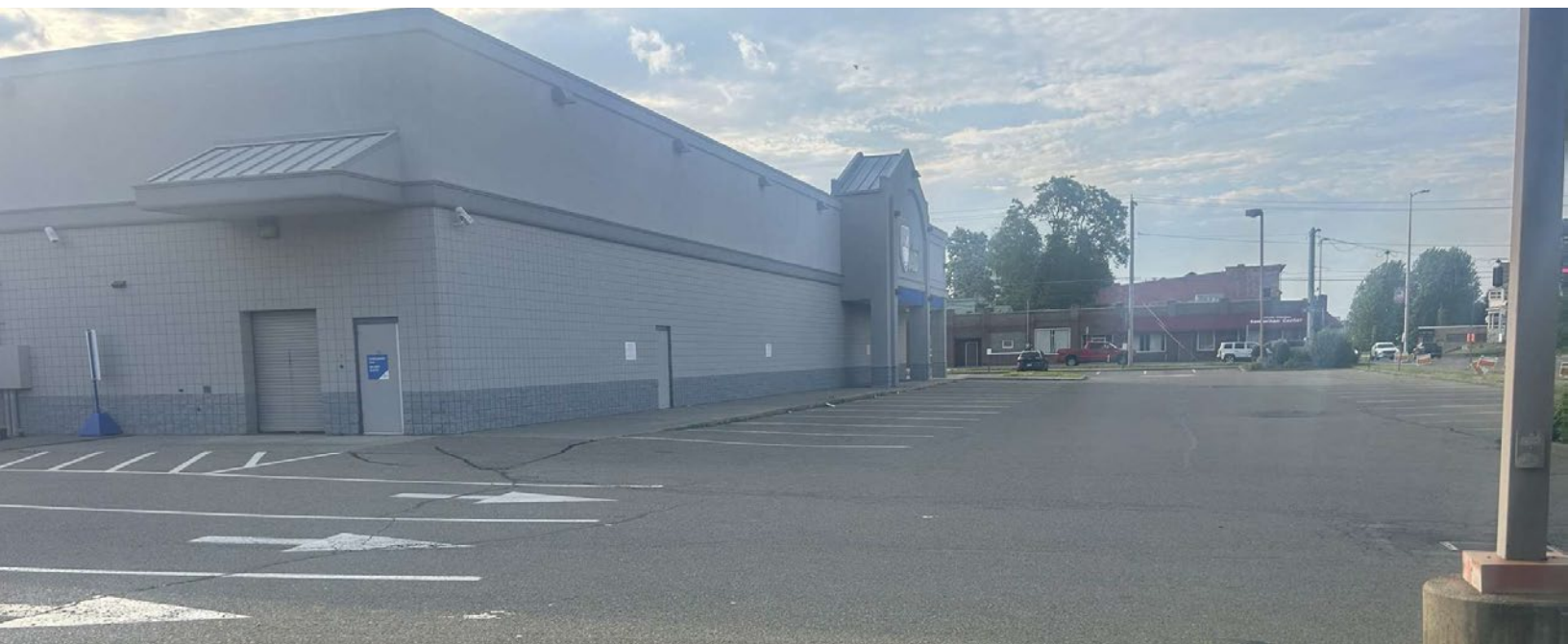
Overhead door for loading
